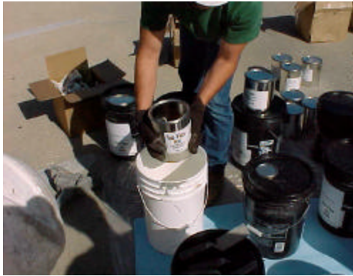
7. Combine tack coat liquid components.
