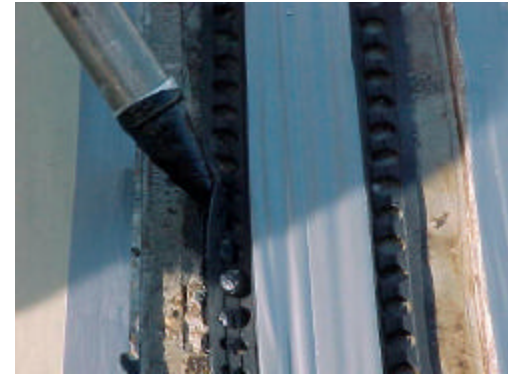
9. Gun tack coat material under wing.
