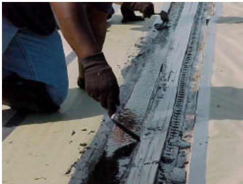
13. Trowel header to a smooth finish.
